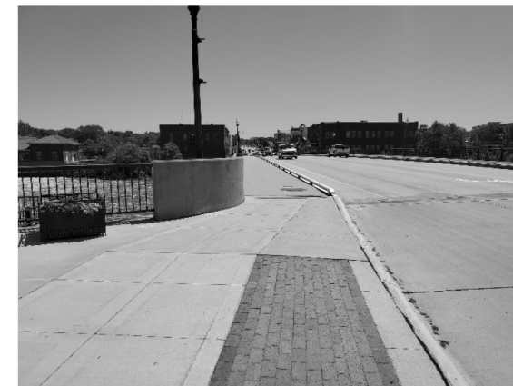
Looking east along IA 3 from west side of bridge
