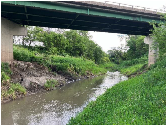
Figure 4: Waterway opening looking upstream, 2024
