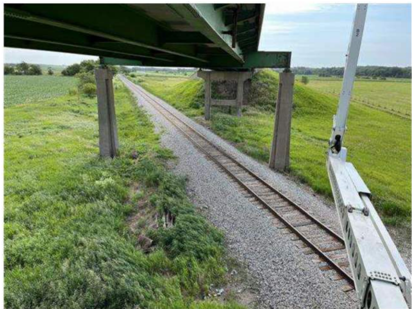
Substructure, Pier 2, facing southeast
