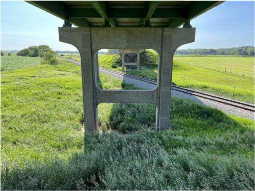
Substructure, Pier 1, facing southeast
