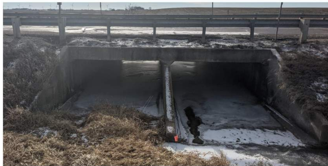
Upstream Face of Culvert
