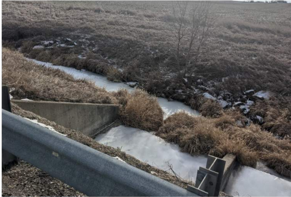
Downstream Channel from Roadway
