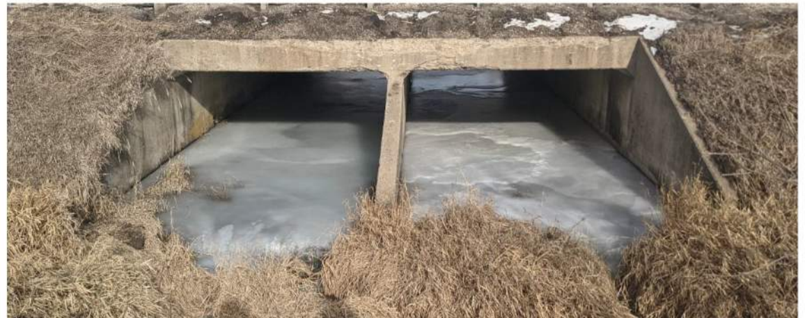
Downstream Face of Culvert
