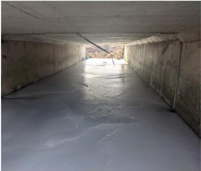
Inside Barrel Looking Downstream
