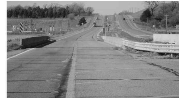
Eastbound bridge facing west
