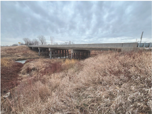
Looking North at Existing Bridge
