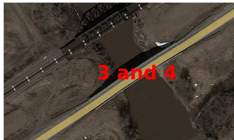
US-30 Crossing the Boyer River
