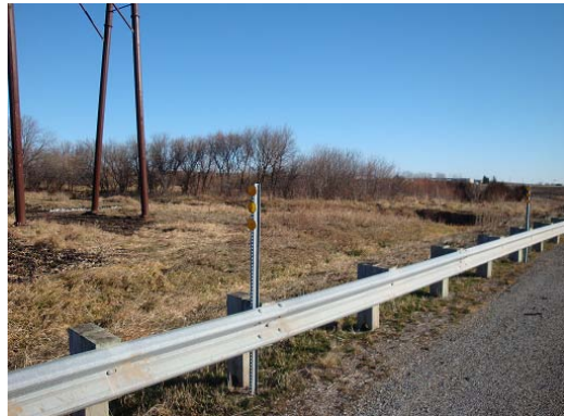
Utility tower on the north side of U.S. 30
