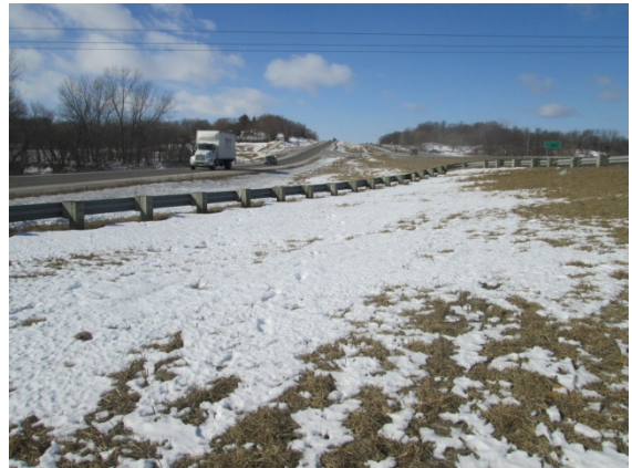
Looking west from west end of bridge.
