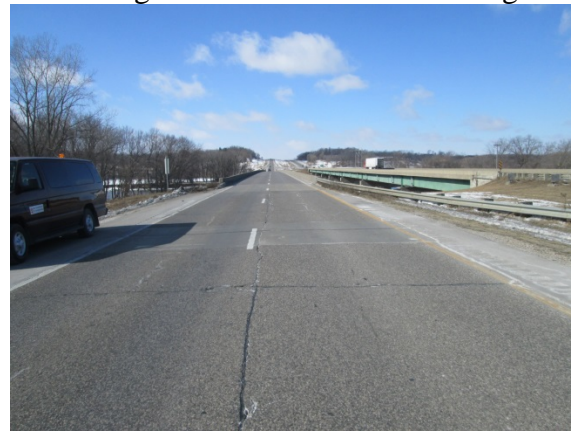
Looking west at the bridge.
