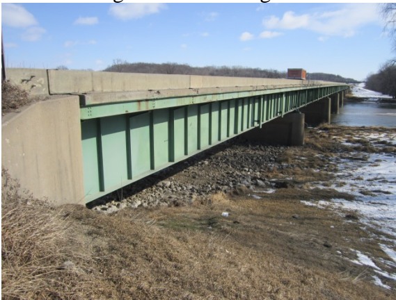
South side of eastbound bridge.
