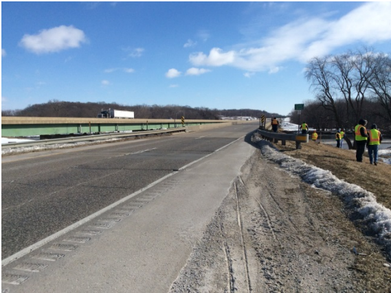
Looking east at the bridge.
