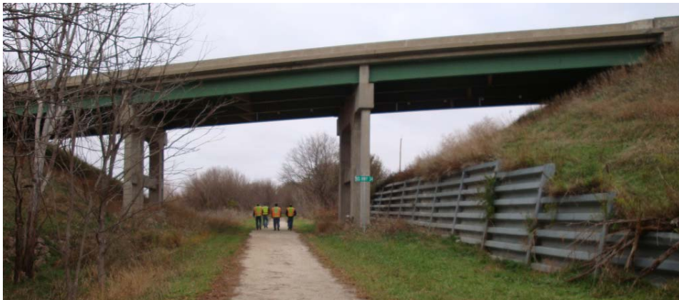
From Wabash Trace Nature Trail under existing bridge looking north
