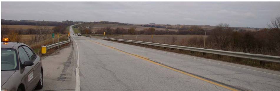
Existing bridge looking west
