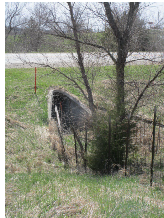
Cattle Pass. Opening within existing clear zone.
