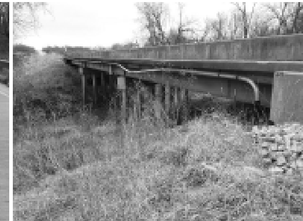
North side of bridge 2021
