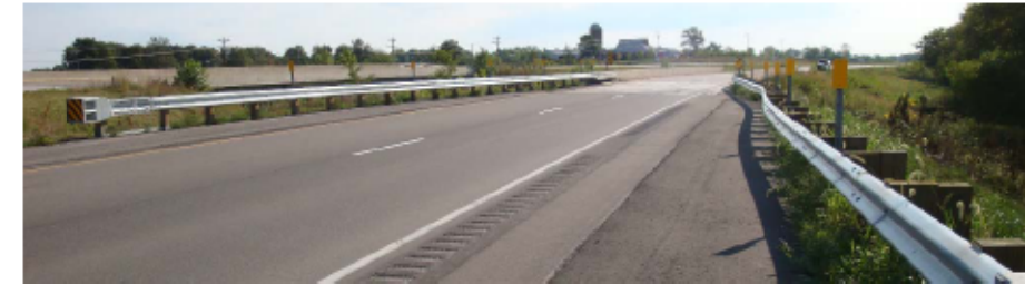
Approaching the eastbound bridge
