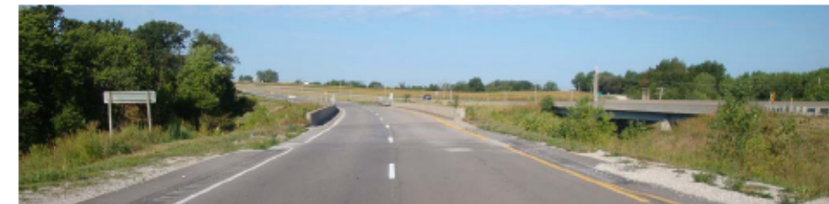
Trailing side of the eastbound bridge
