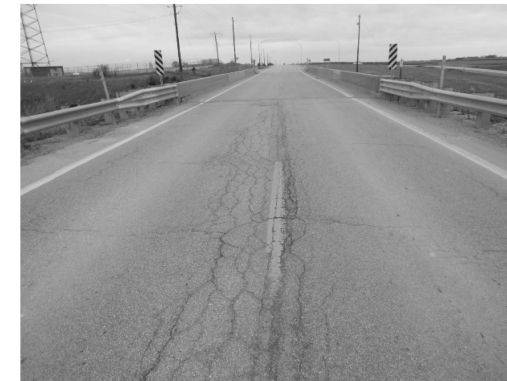
US 59 looking North
