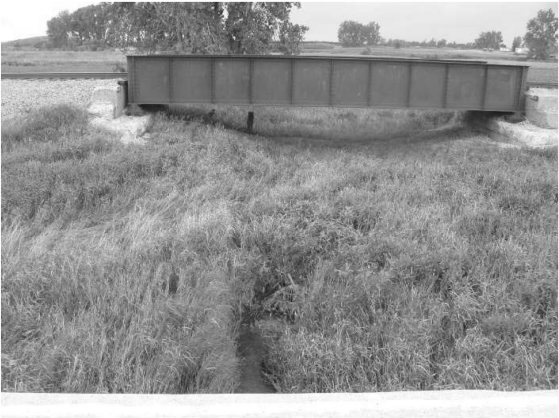
Downstream Including Railroad Bridge
