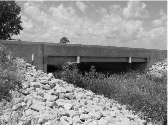
Right Profile of bridge
