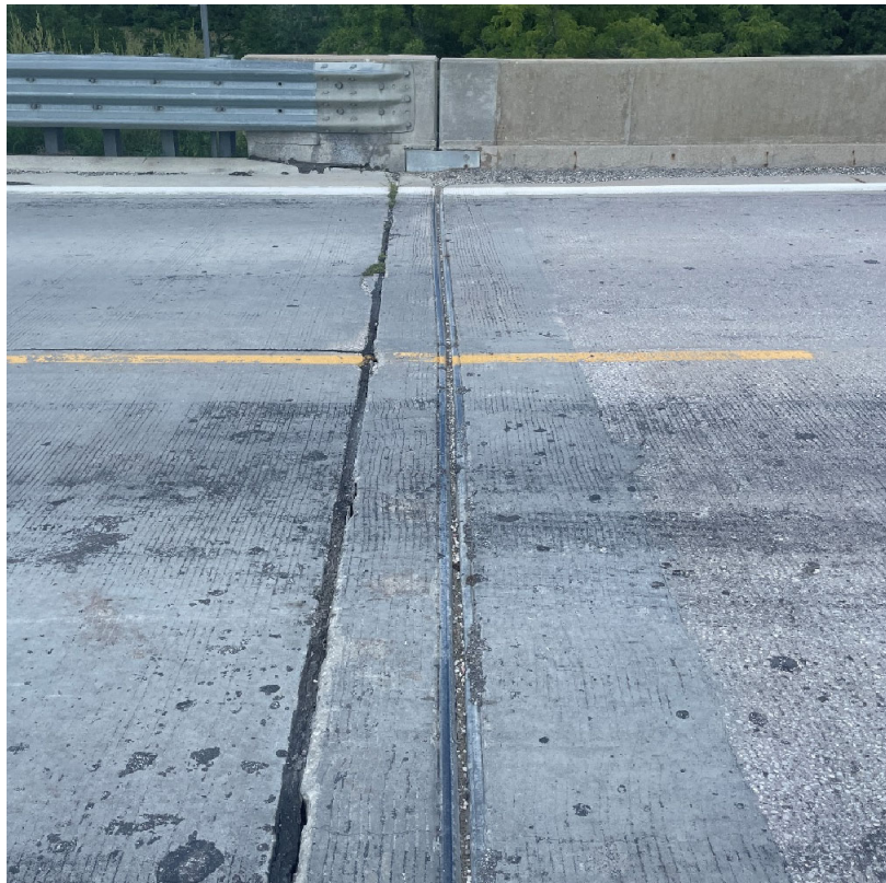
Image 5: Near Abutment Joint (Looking North)
