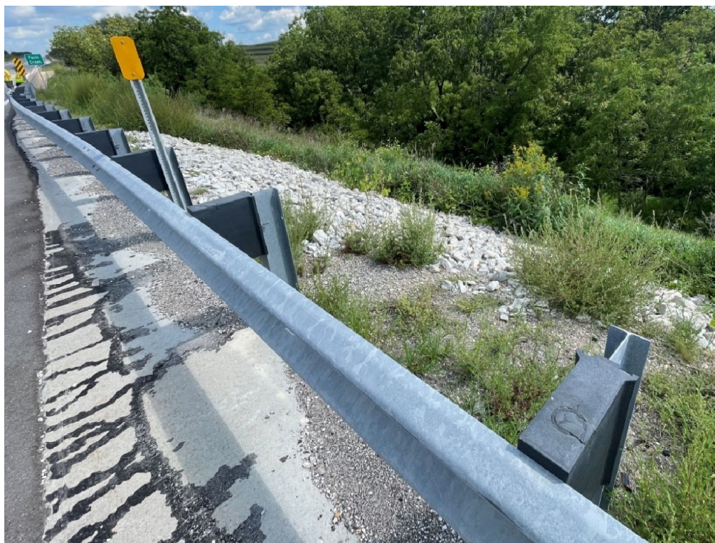
Image 2: Near Approach Slope Protection (South Side)
