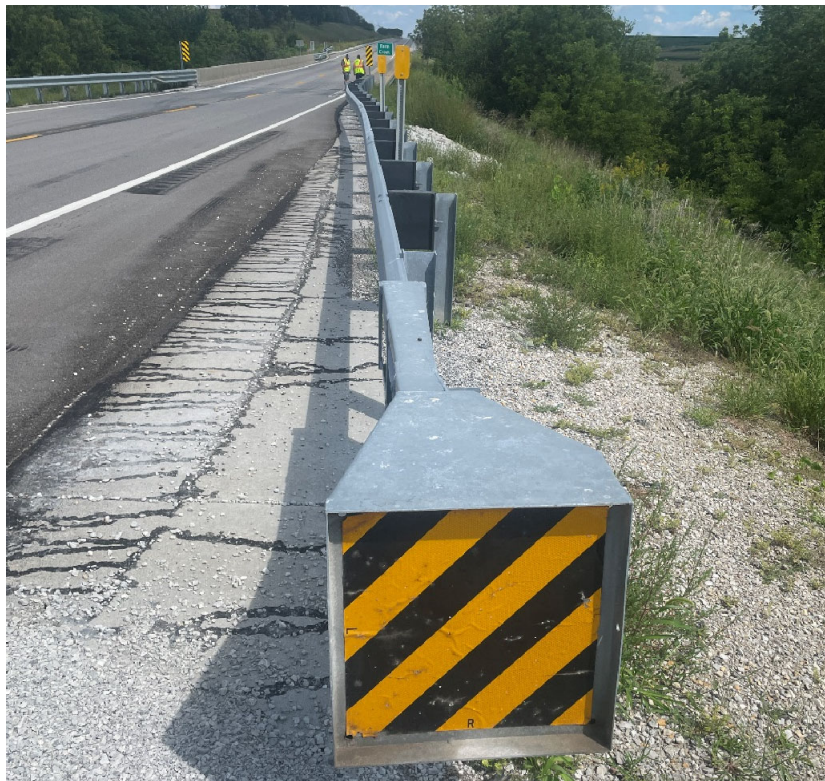
Image 1: Near Approach Guardrail (South Side)
