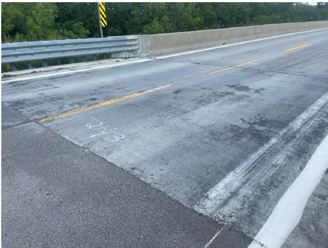
Image 3: Near Approach (Looking North)
