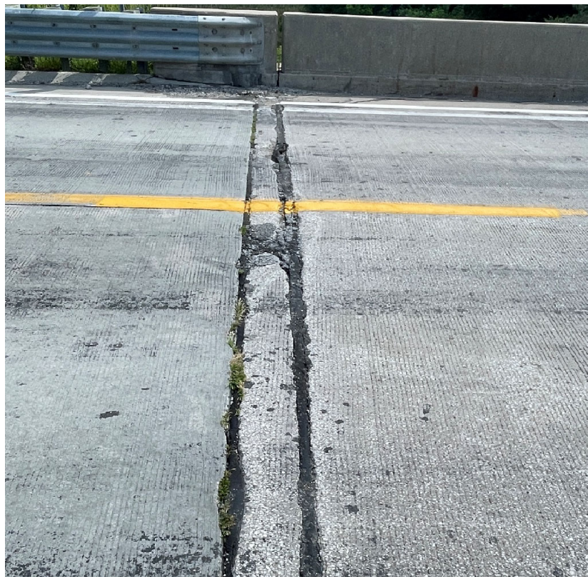
Image 6: Far Abutment Joint (Looking South)
