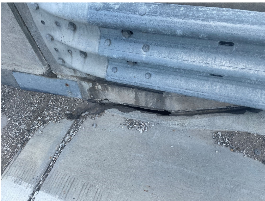
Image 4: Near End Barrier Seal (South Side)
