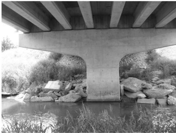
Pier 1 far face
