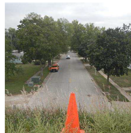
Roadway through (right)
