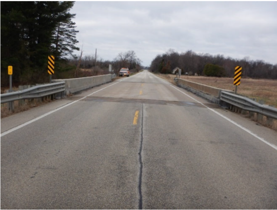
Figure 3: Against route facing west, 2024
