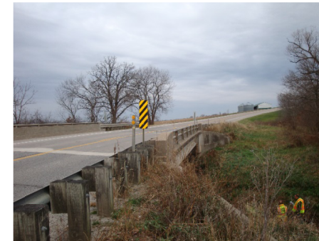
Sight distance looking west
