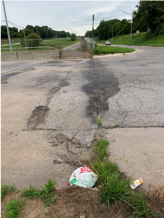
South approach looking east
