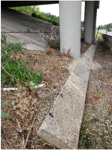
Toe of south abutment concrete slope protection
