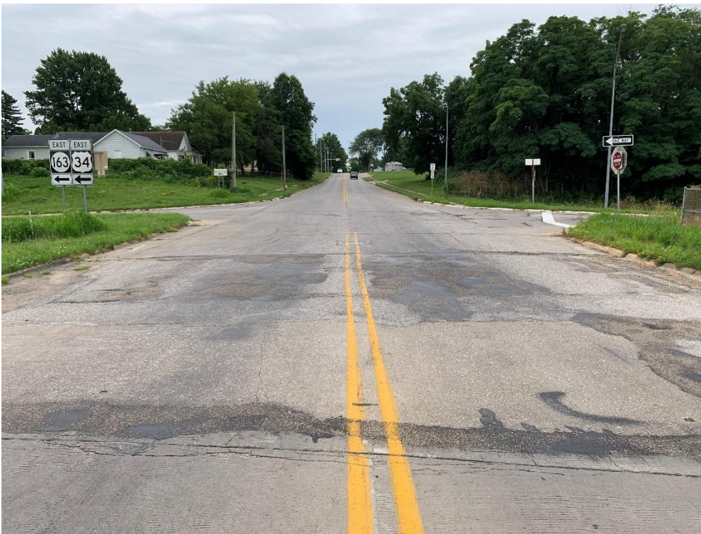
North approach looking north
