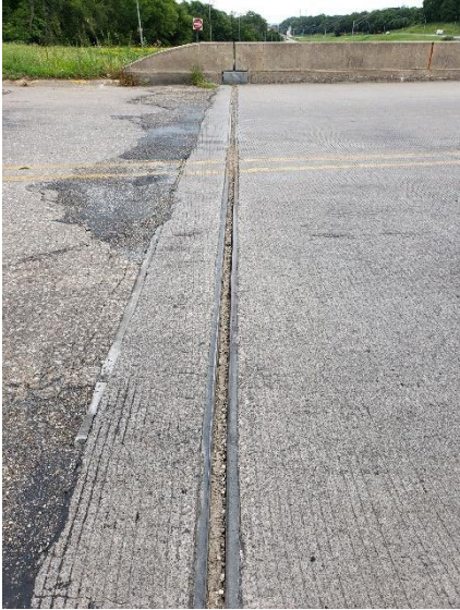
North abutment joint
