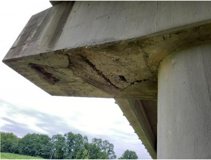
East side of pier 3 overhang
