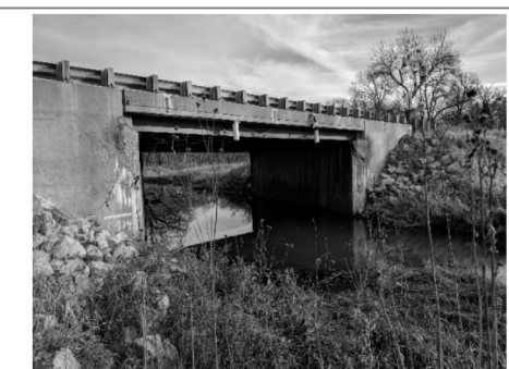
Looking north at bridge
