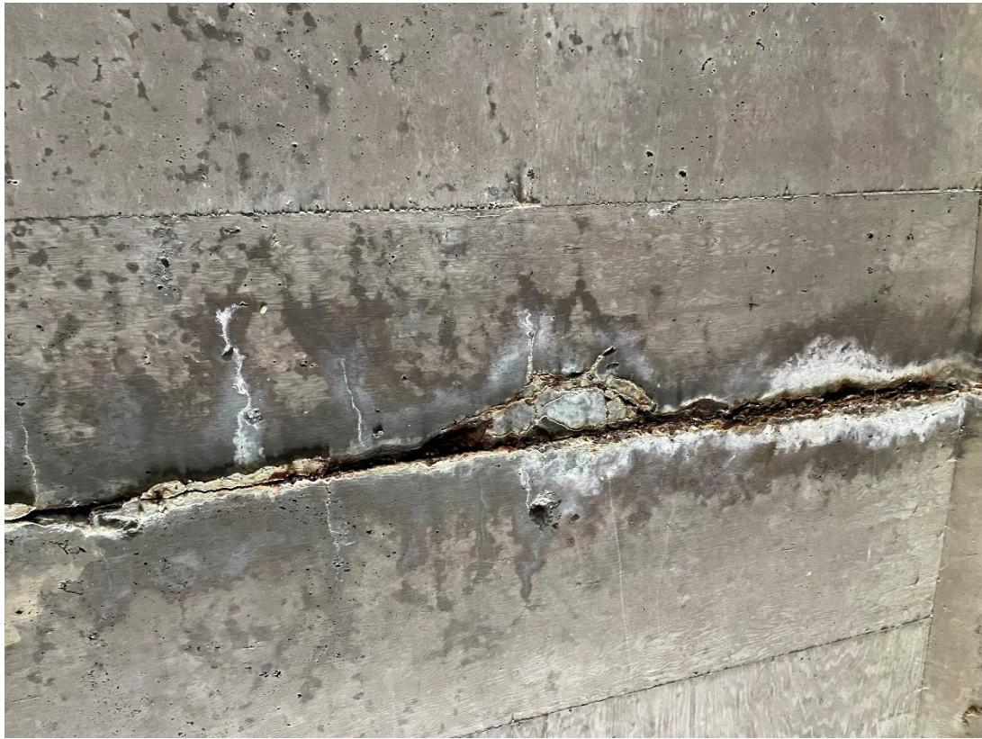
Typical Top Slab at Construction Joint
