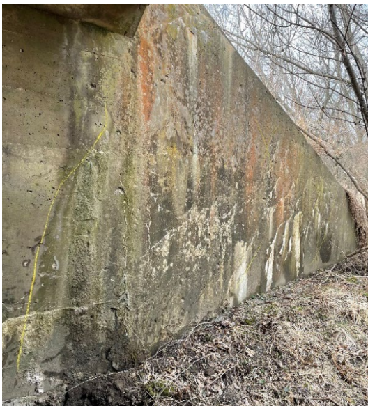
Deterioration at Southwest and Southeast Wings
