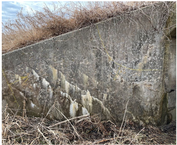
Deterioration at Southwest and Southeast Wings
