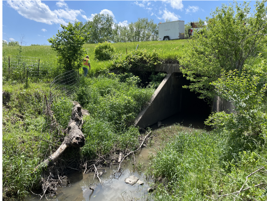
Culvert Headwall View (East Headwall looking West)
