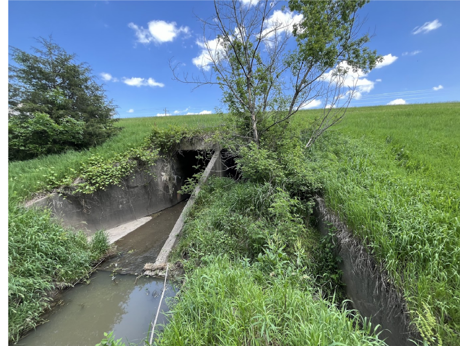
Culvert Headwall View (West Headwall looking East)
