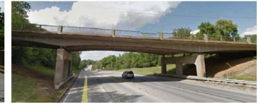
Bridge as seen from IA 149
