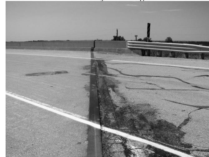
Far abutment joint looking south.
