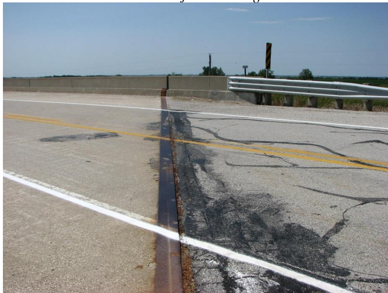
Far abutment joint looking south.
