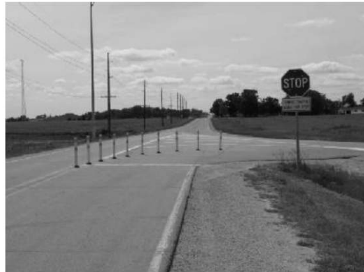
Alternative 1 New pavement markings, stop sign and tubular markers For Westbound Traffic on 55 th Street
