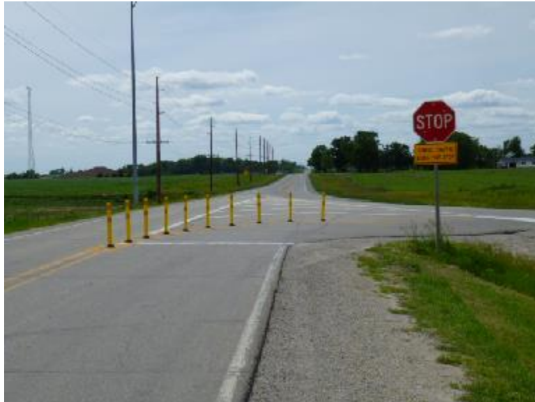
Alternative 1 New pavement markings, stop sign and tubular markers For Westbound Traffic on 55 th Street
