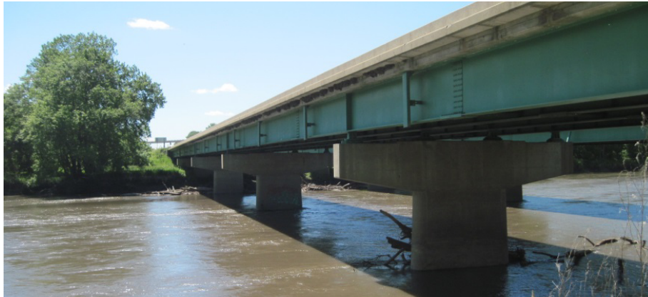
I-80 Eastbound at North Raccoon River
