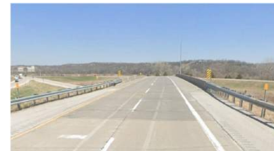
Northbound I-29 facing northeast
