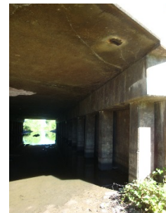
Below looking West
