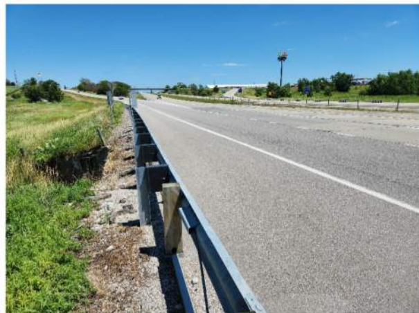
WB roadway looking E at N end of culvert
