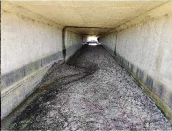
Silt in west barrel
