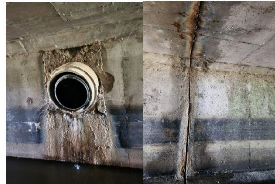
Storm sewer in west wall
