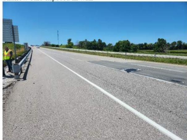
EB roadway looking W at S end of culvert
