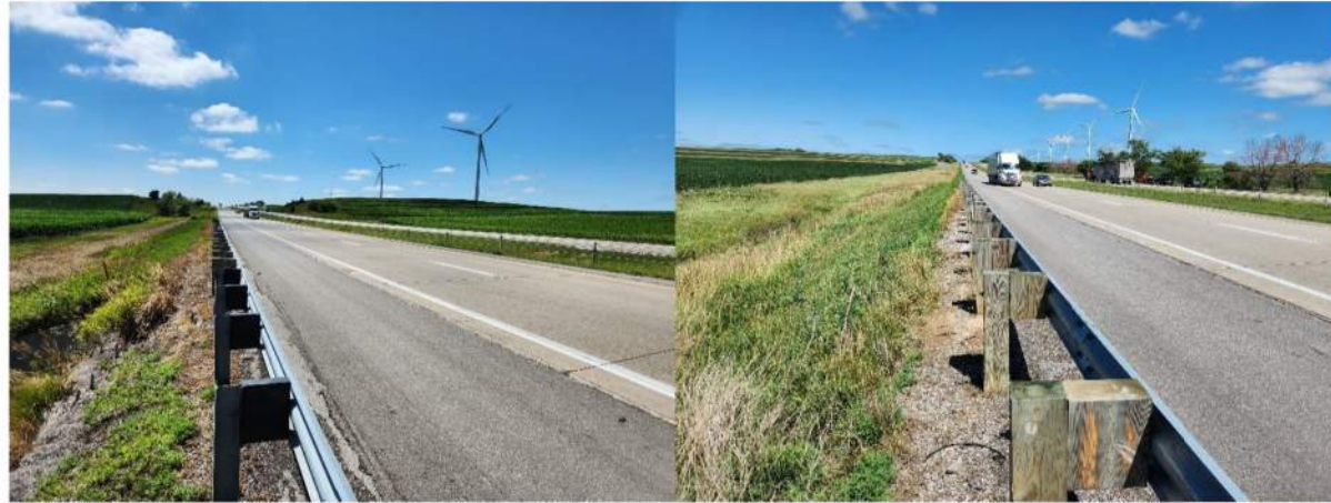
EB roadway looking W at S end of culvert
