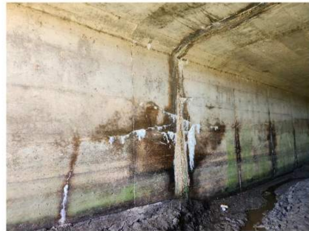
Typical construction joint condition
