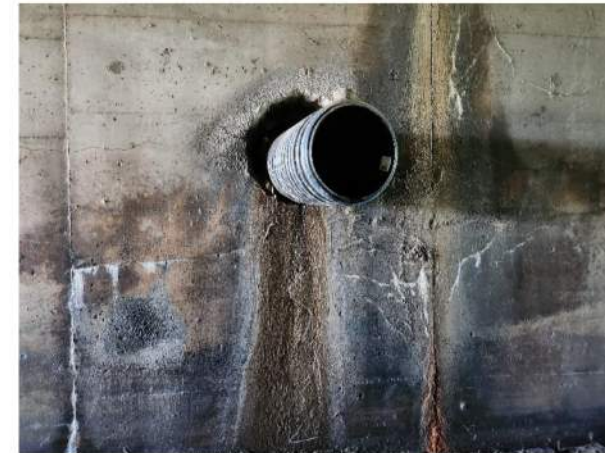
Storm sewer in west wall
