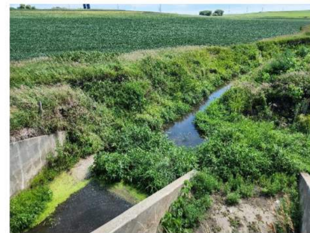
Channel downstream (2' drop)
