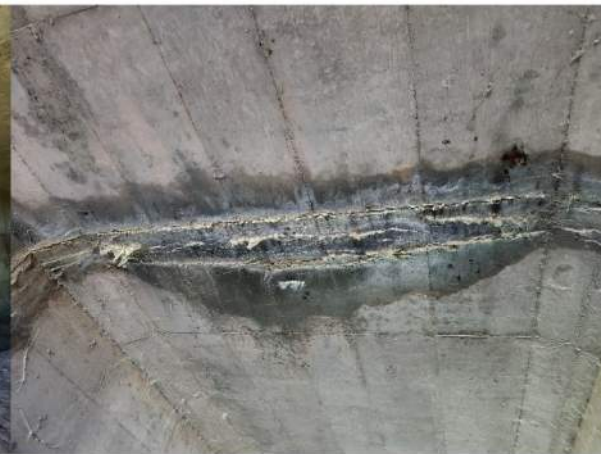
Typical slab construction joint
