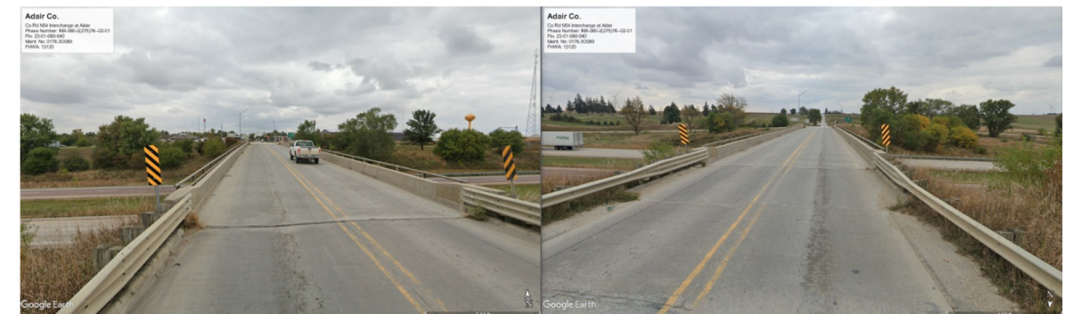
Northbound Co Rd N54
