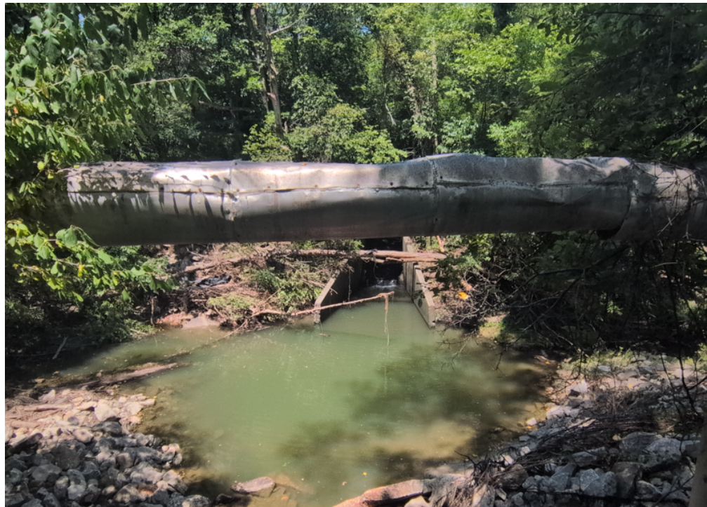
Photos showing sanitary sewer at downstream end of 7' x 10.5' arch culvert Sta. 2535+35
