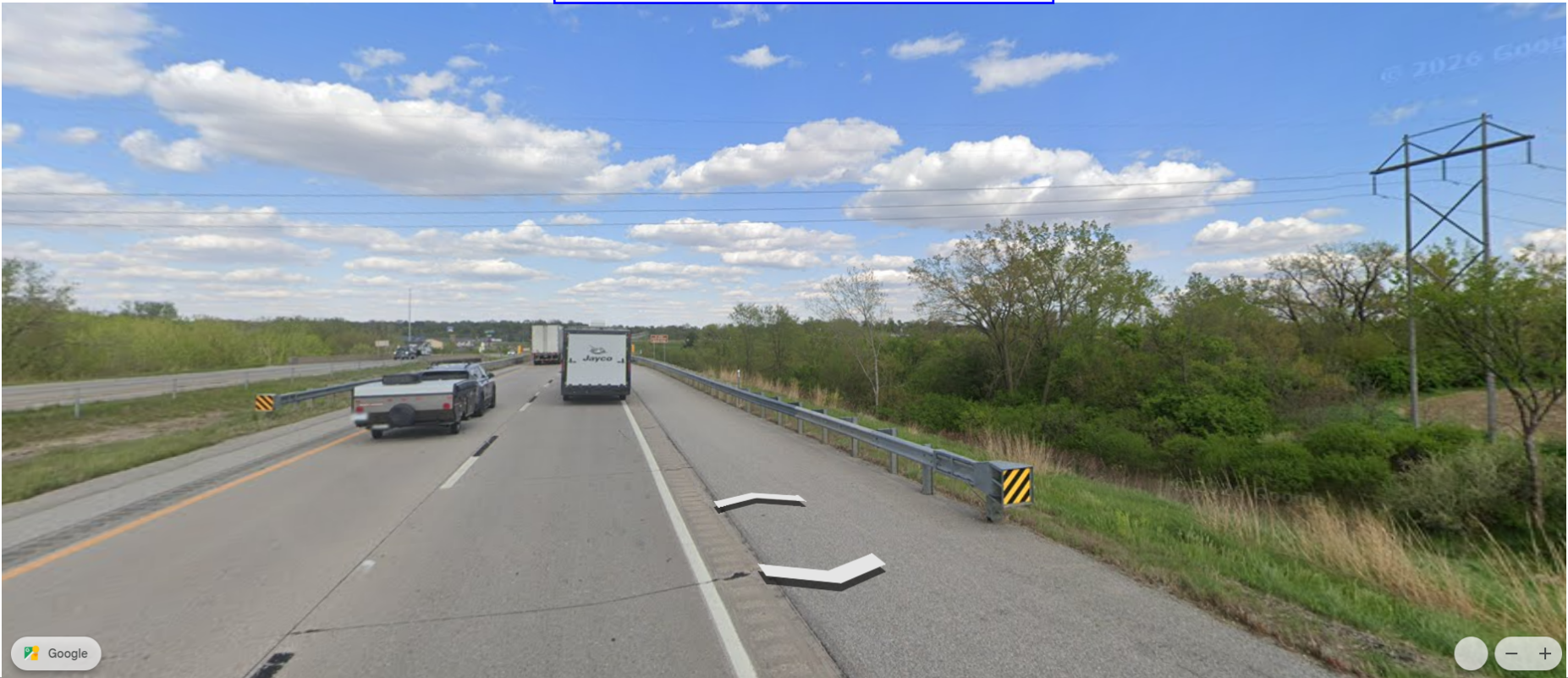
Electric transmission line west of bridges
