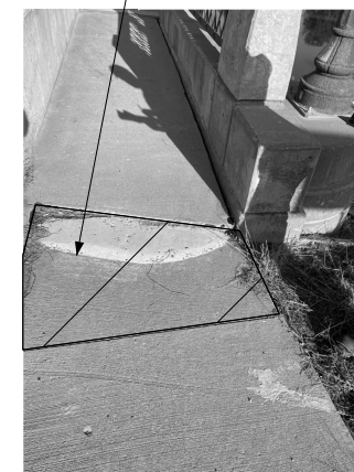
Sidewalk Removal and Replacement at Southeast Corner
