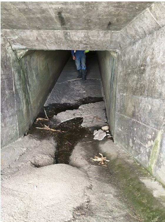
Inlet end of the culvert
