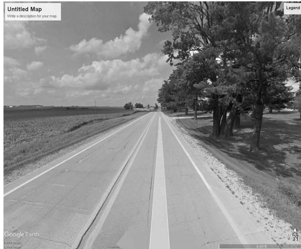
Figure 1: Iowa 13 Looking North, Showing Pavement Joints and Trees in Clear Zone
