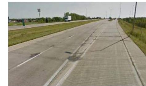
WB exit ramp at US 63
