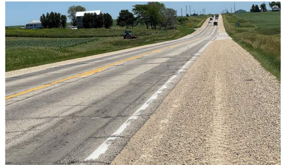
Figure 1: Existing granular shoulders eastbound lane
