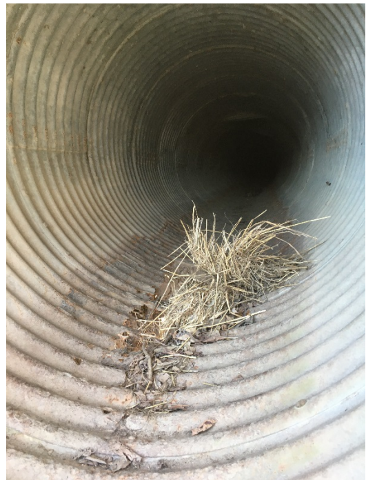
42" CMP - Looking West
