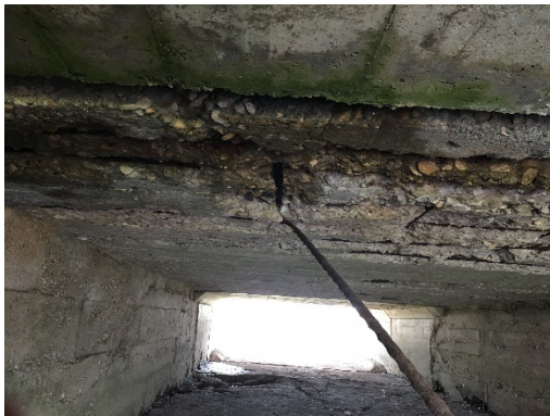
Condition of Existing Culvert
