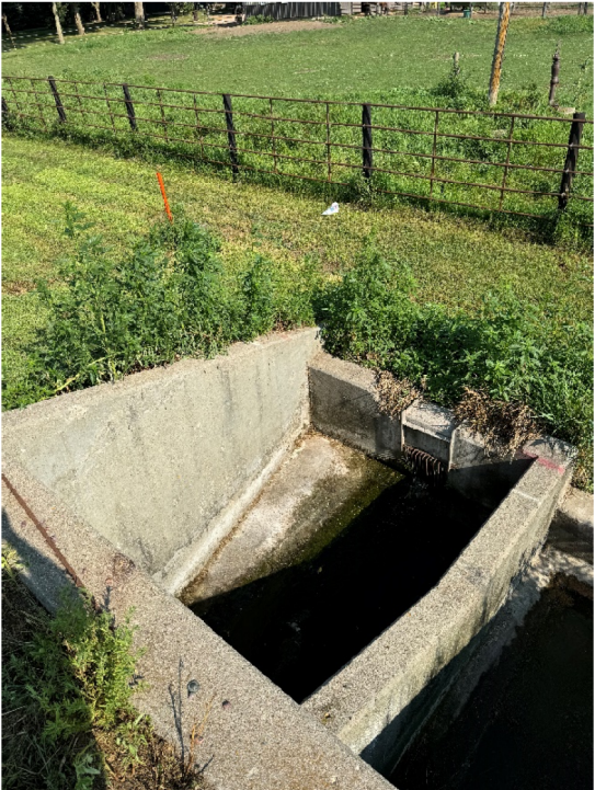
Inlet Weir Structure.
