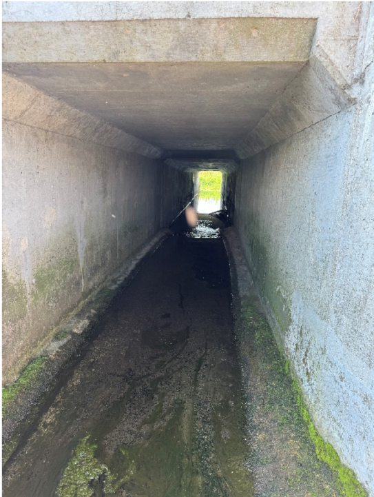
Left Barrel looking South.
