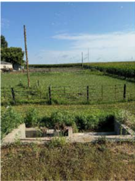
Inlet Looking North
