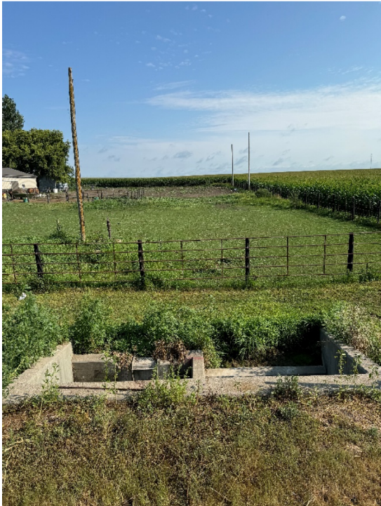
Culvert Inlet and Weirs looking North.
