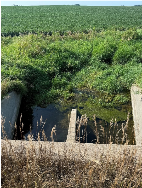
Culvert Outlet looking South.
