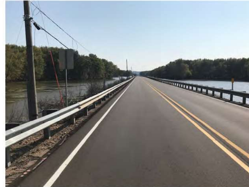
Attachment 1 – North end of alignment looking south
