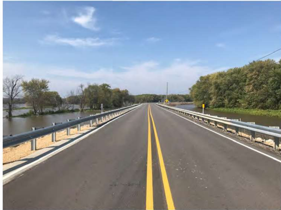
Attachment 1 – Looking north at south project limits
