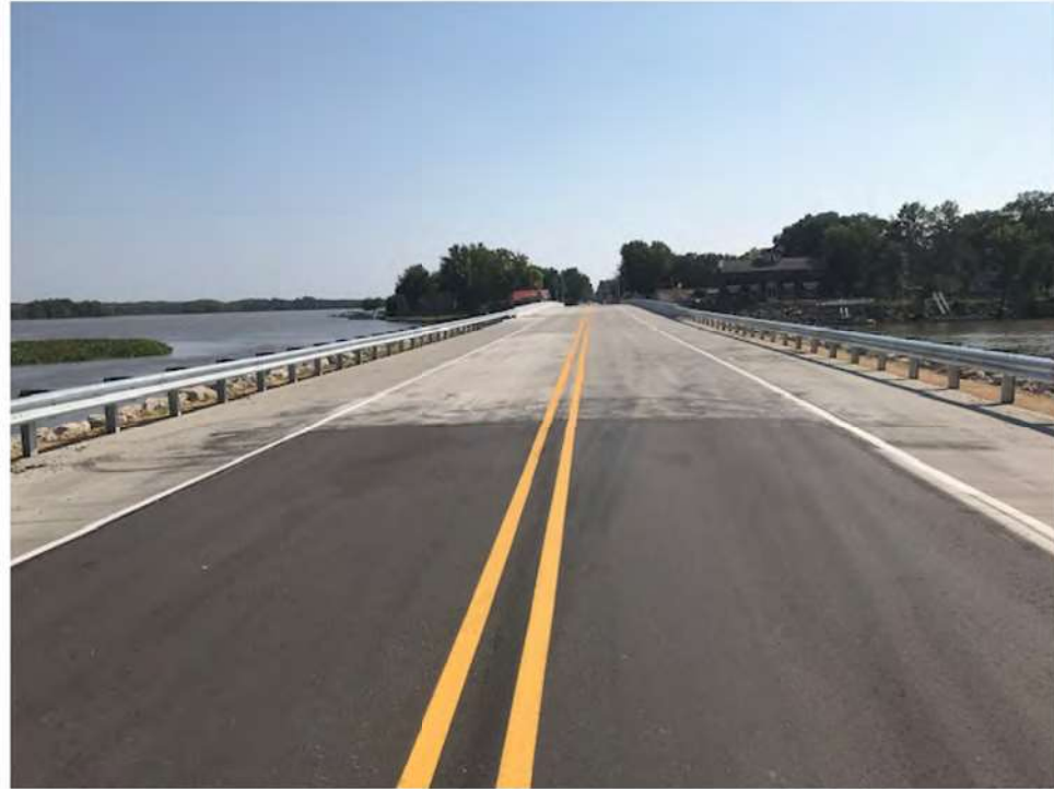
Attachment 1 – Looking south at south project limit towards overflow bridge
