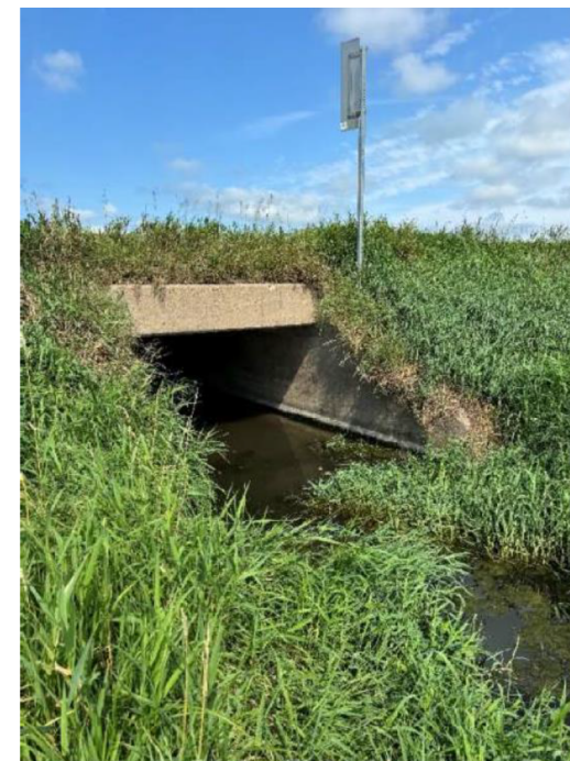
Upstream Face of Culvert
