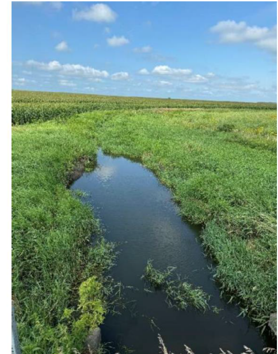
Downstream Channel from Roadway
