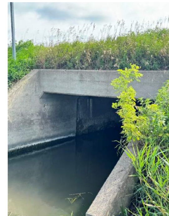
Downstream Face of Culvert
