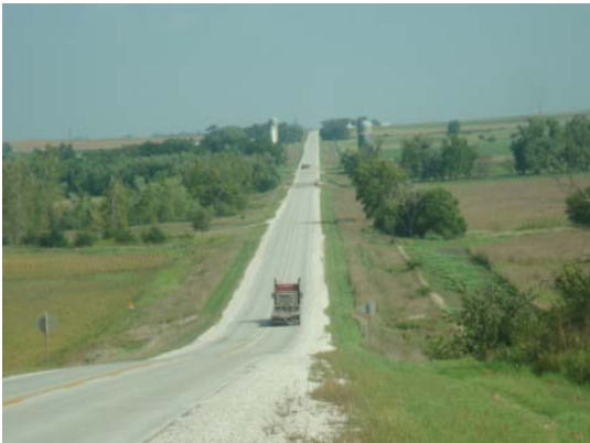
South end of project looking north
