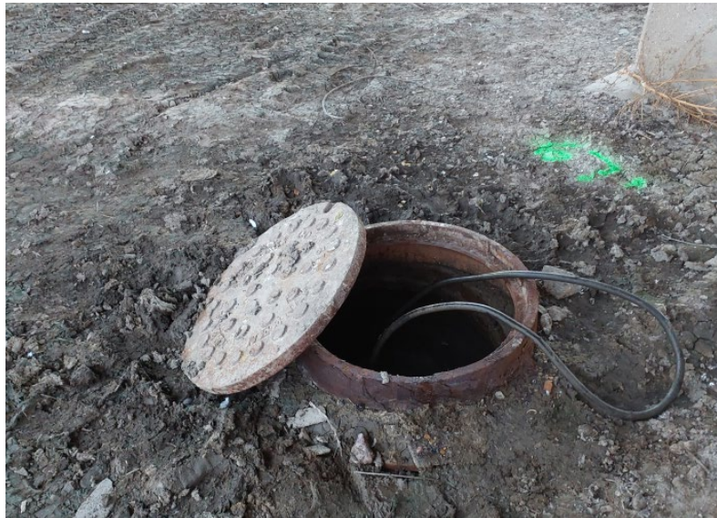
Figure 2. Electric cable observed in Structure 674
